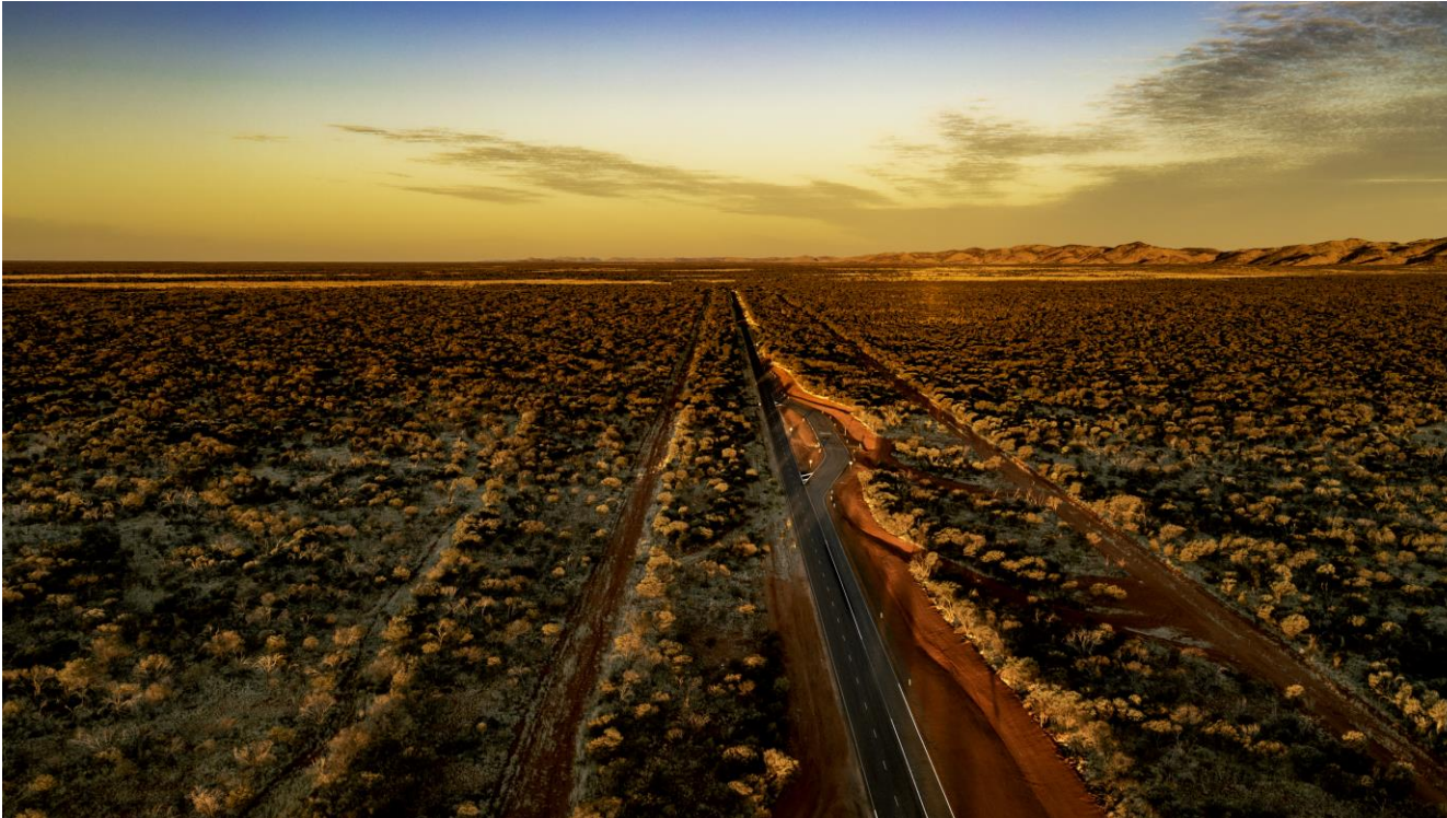
Figure 20: Aerial photograph of Tanami Road upgrades
